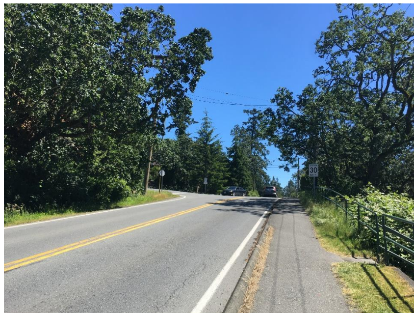
Example of a sidewalk on Burnside Road W where there is minimal protection from vehicle traffic along with grass encroaching on pedestrian space
