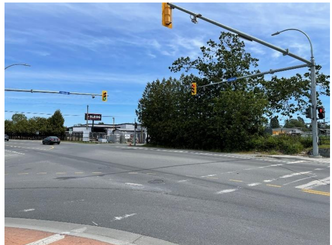
Example of a poor pedestrian crossing at Admirals and Hallowell intersection (faded markings, crossing distance). There is also a lack of sidewalk connectivity.
